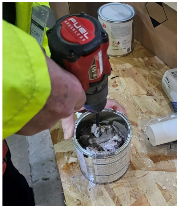
Plate 12 – Adhesive Mixed using Plastic Paddle Attached to Drill
