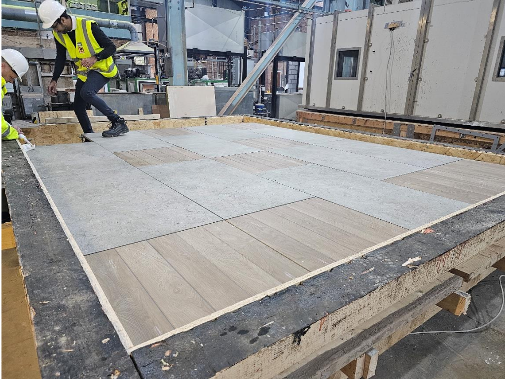
Plate 15 – Completed Test Sample
