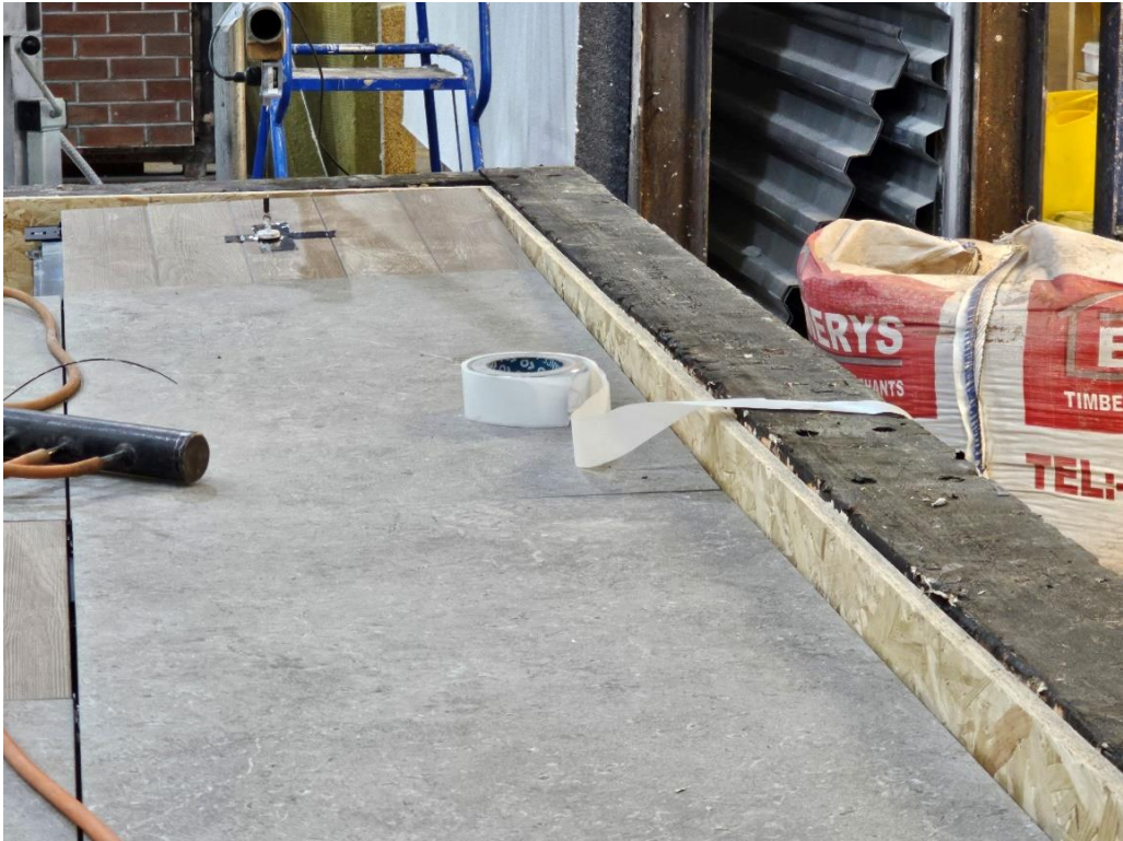
Plate 20 – Tiles Lifting During Load Testing of A-PED-JOIST Section
