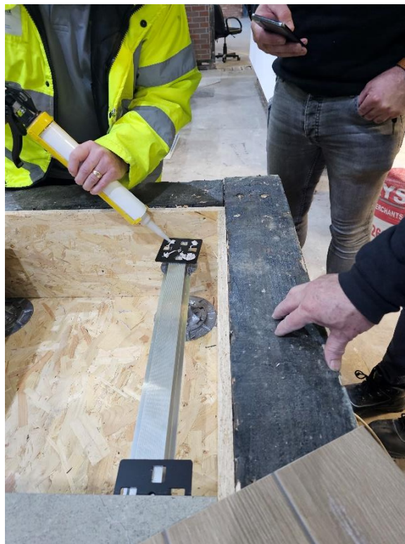
Plate 14 – Adhesive Applied to Tile Spacer/Pedestal Tops
